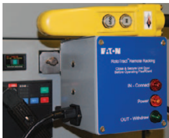
FlashGard LV MCC Remote Racking Device
