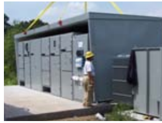
Deposit on Base Enclosure
