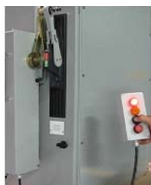
Ampgard MV Starter ISO Switch Operator
